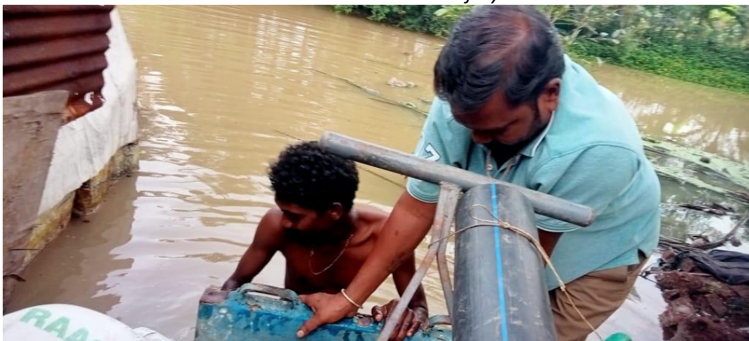
Photo 8: Community members and volunteers supporting emergency restoration efforts in flood-affected areas.
